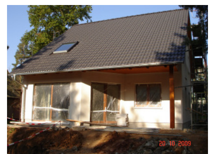
Bauvorhaben in Chemnitz
