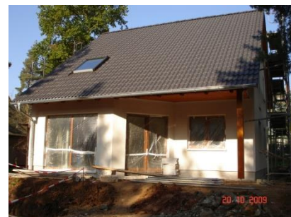
Bauvorhaben in Chemnitz
